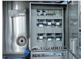
Valve terminals CPV can be positioned inside the control cabinet using wall or DIN rail mounting.
