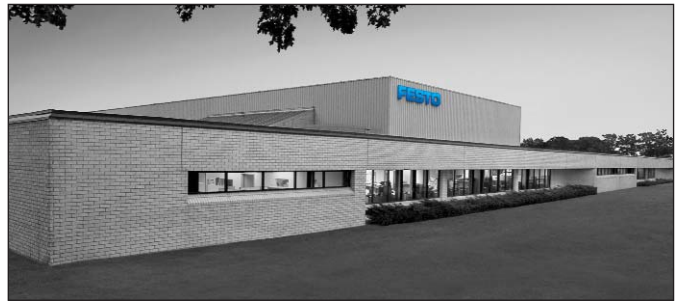
East: 395 Moreland Road, Hauppauge, NY 11788
