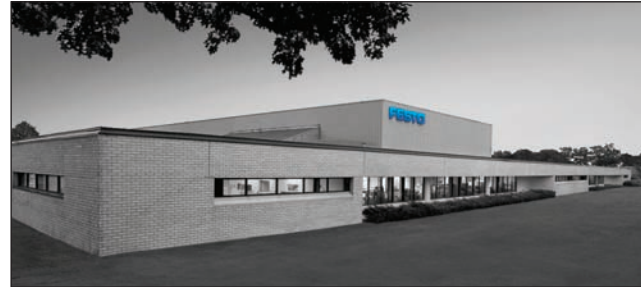
East: 395 Moreland Road, Hauppauge, NY 11788
