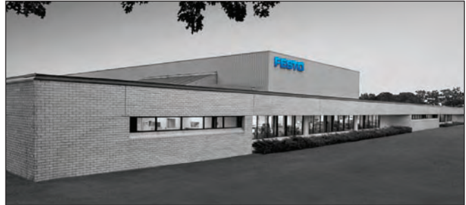
East: 395 Moreland Road, Hauppauge, NY 11788
