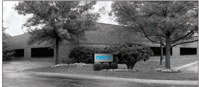
Central: 1441 East Business Center Drive, Mt. Prospect, IL 60056
